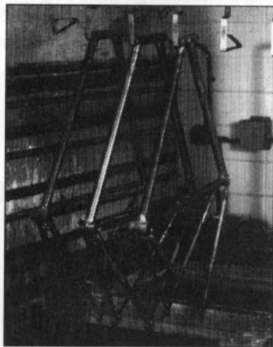
Frames are dipped into a nasty, caustic bath for anti-rust treatment inside and out. Then they're primed, painted, decaled, clear-coated, and further treated with FrameSaver.
